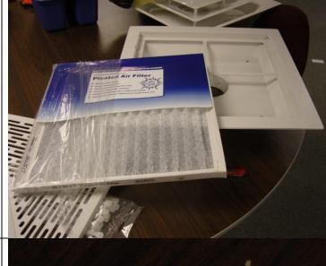
Check for the proper filter air flow direction. Begin the installation by preparing and assembling the exhaust grill to the flex ductwork. The filter is designed to have a specific orientation which can be identified by an arrow or something similar to Figure 3.
