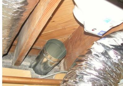
Fans can be fit between floor joints even in very tight cellings and then mounted with the supplied bracket into the drop ceiling as well.
