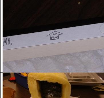
Pull back the insulation on the flex duct and tightly seal the duct to the grill. This was done by using aluminum tape to adhere the two together. Then, to keep it securely in place and to help reduce any strain on the attachment when being installed, a large zip tie was added on top.
