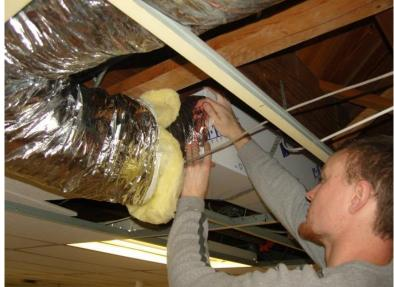
After the ERV is installed and all the duct work is run, retain a skilled masonry contractor to make penertattions in the exterior concrete wall for exhaust air. Wood framed walls can be penetrated by a hole saw.
