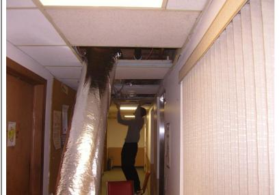
Mount the Energy Recovery Module in the drop ceiling or designated area. Most Energy Recovery Modules are difficult to install overhead and in tight spaces because of their weight and size. That is why for this application BPE-XE-MIR 200 was optimal. It is made of Polypropylene and is long and narrow.
