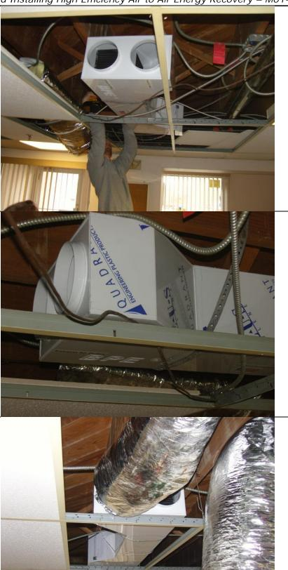
Seal the inside lining of the duct work with aluminum tape. Then secure the entire duct work with a zip tie over the insulation, aluminum tape and ERV lip the same way as connecting the duct work to the filter grill.
